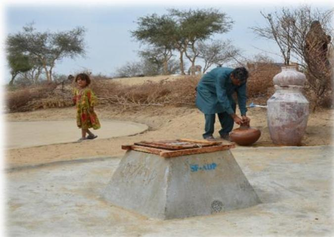
During reporting period construction of village level structure, small household level Nadi pond cisterns (underground tanks) are also part of village level rainwater harvesting system. The internal shape of the Nadi pond allows it to be constructed using a very thin lining of cement and sand mortar. These Nadi ponds catch the monsoon rains via a small saucer shaped
