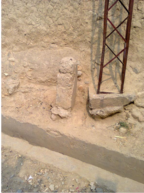
Figure 5: A non-functional tap stand of previous water system
