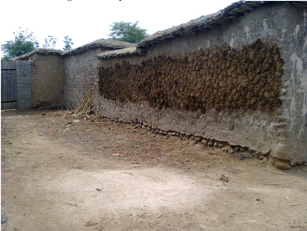
Figure 8: A possible site for hand pump installation
