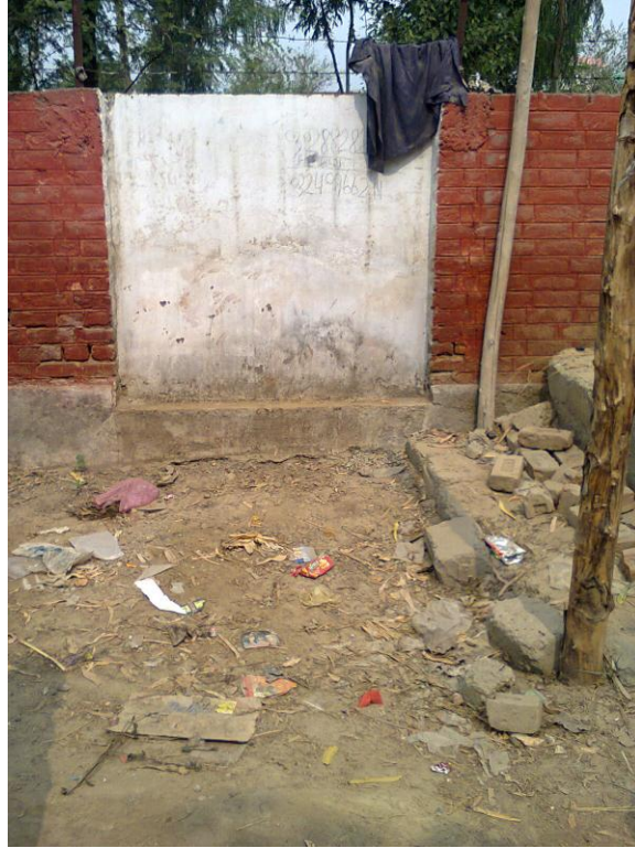
Figure 11: A possible site for hand pump installation
