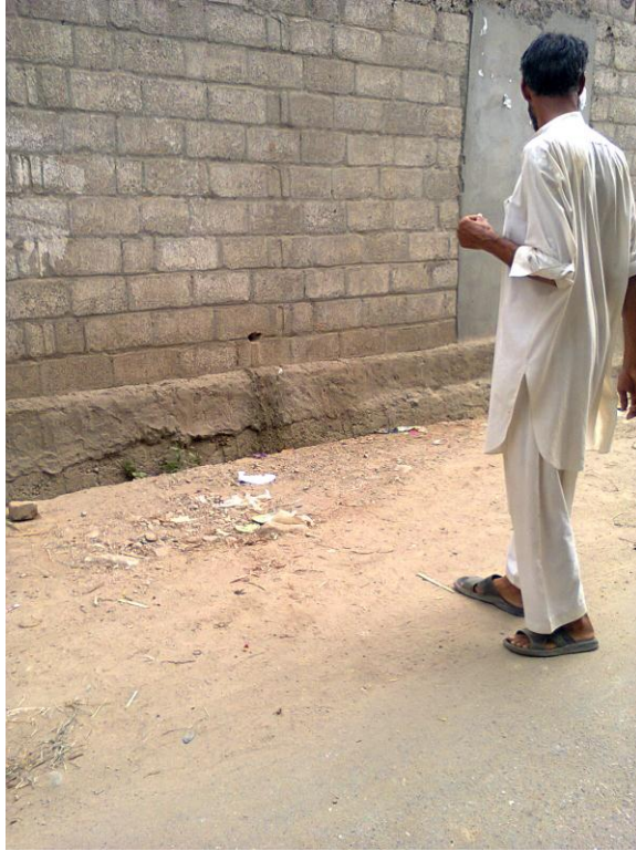
Figure 9: A possible site for hand pump installation
