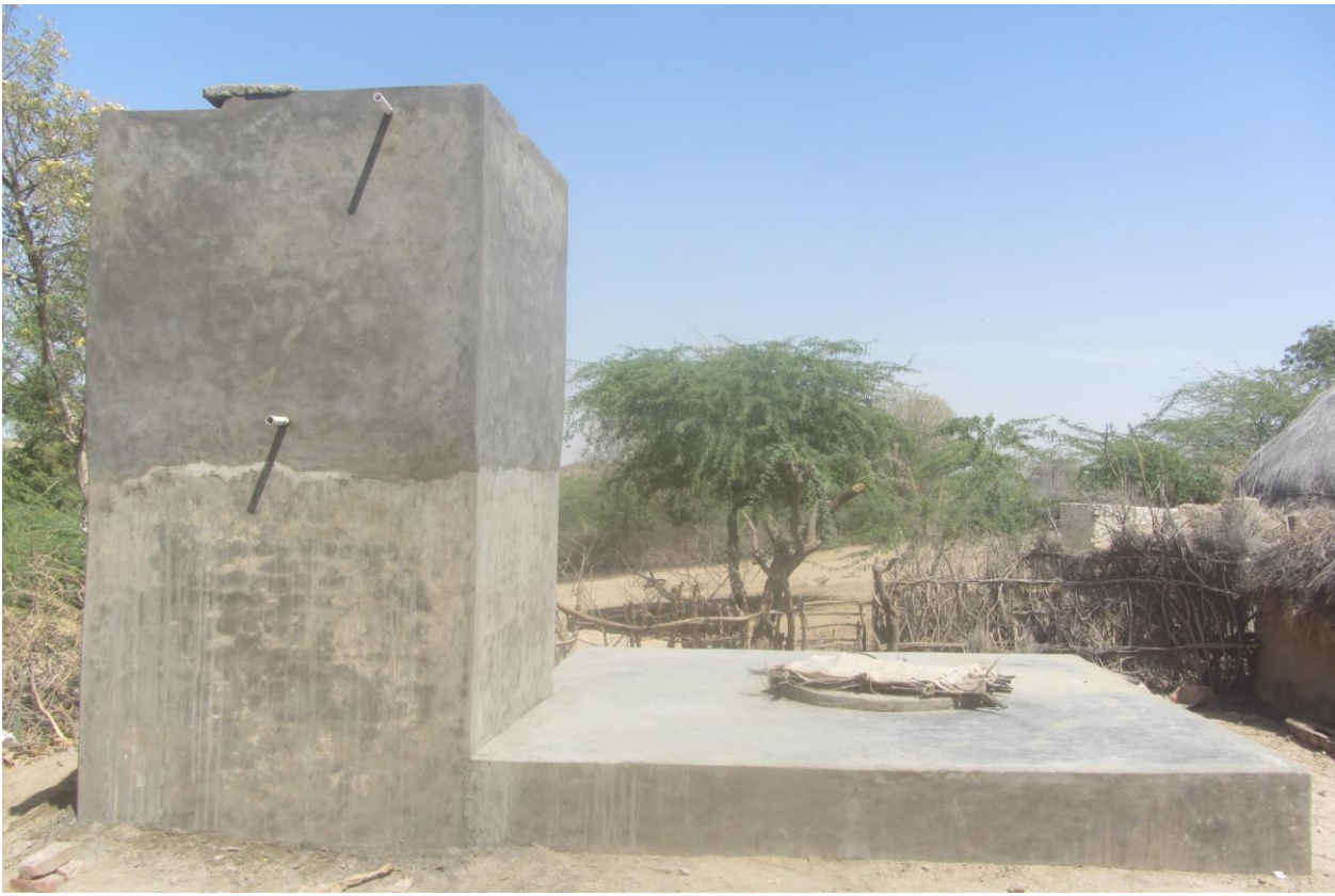
Platform and dug well modification completed
