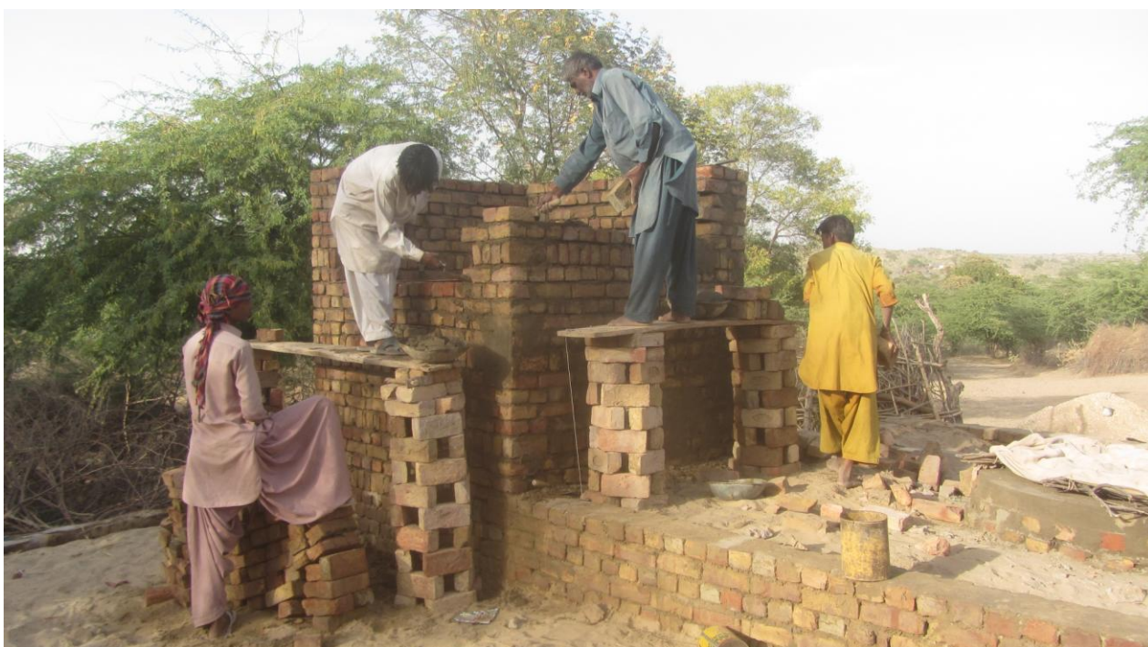
Constriction of overhead tank
